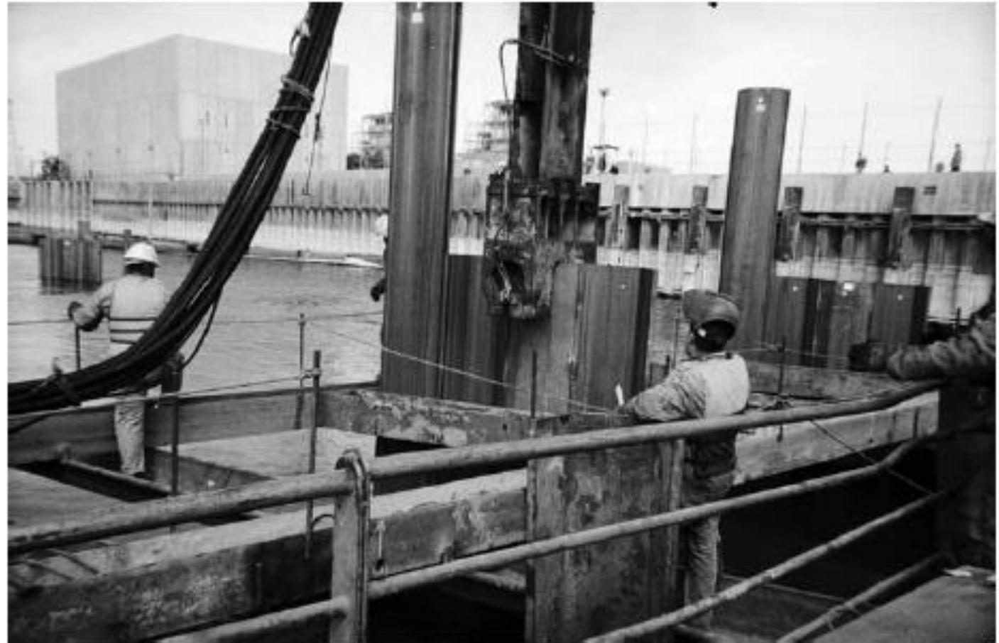
**Figure 6-4.** Vane installation at Kuraimat Power Station, the Nile River, Egypt, 2007. Photo shows sheet-piles being driven in a template that controls vane orientation. Intake is in the background of the photo. Courtesy of Adnan M. Alsaffar.
